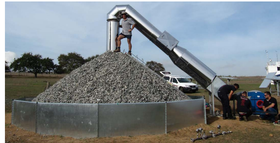
Rock Bed Thermal Storage: Construction Photos
